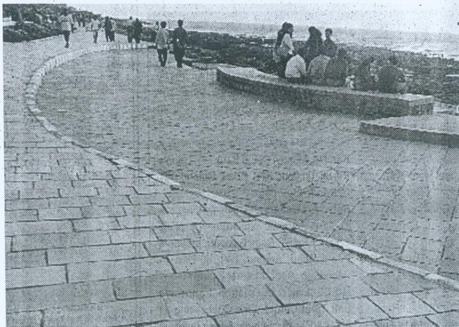
Bandra Bandstand after the redevelopment work
